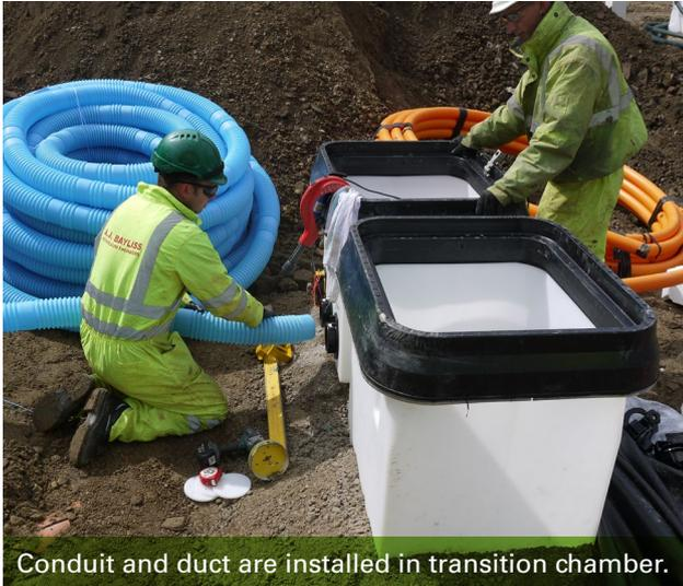
Conduit and duct are installed in transition chamber.
