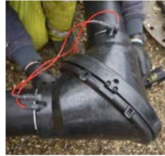
Welding the Gemini Fitting in one process with jumper leads.
