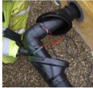
Welding the primary elbow.
