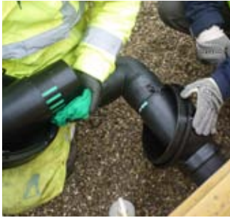
Preparing the elbow assembly.
