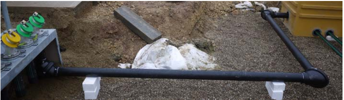
The final fill line in place.
